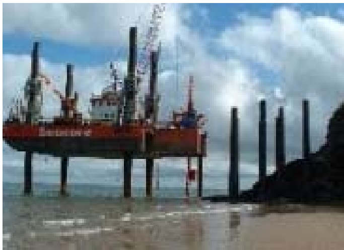
A Seacore platform. Photo: Fugro Seacore
